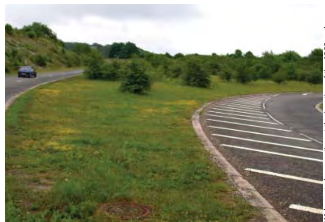
Wide central reservation at the junction of the A303 and A3057, of potential value for wildlife. A Spalding
